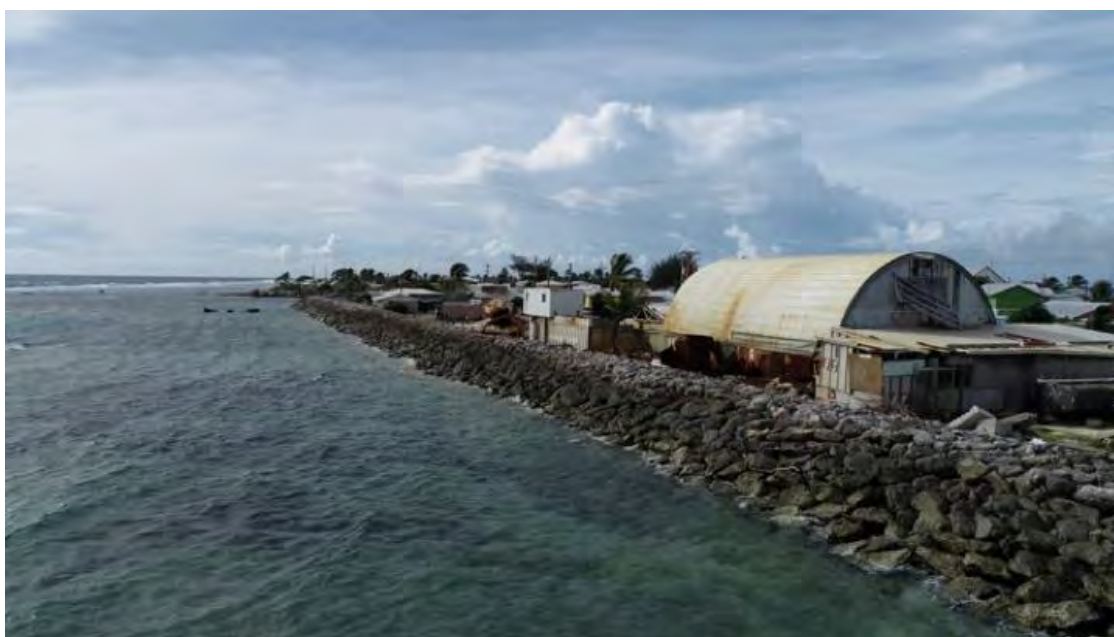
Figure 2-8: Existing Revetment on Ebeye
